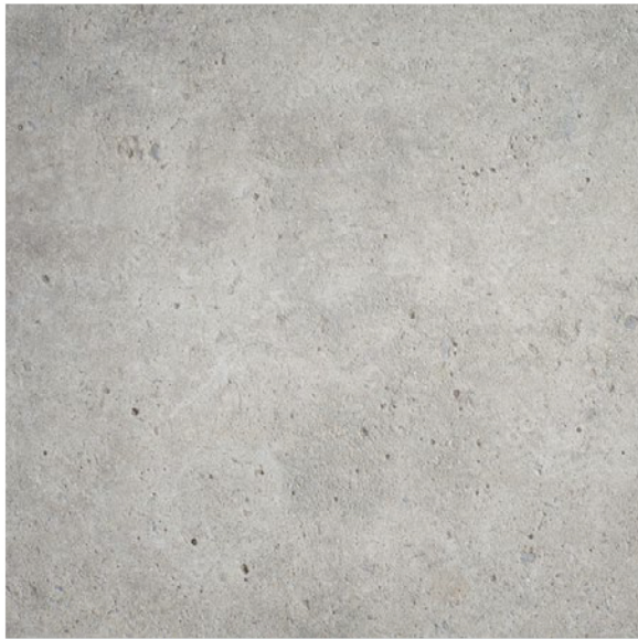
Cast in place concrete foundation
