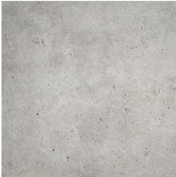
Cast in place concrete foundation
